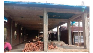
First floor of Children's Residence
